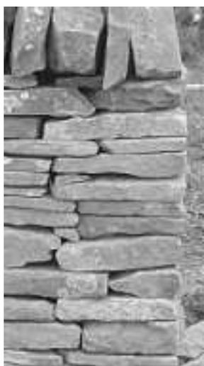
The sandstone end left (seen in part 1), demonstrates the problem that can easily occur – in this instance the lower of the 2 sets of joints has been created by placing short runners on wide broken ties, whilst the upper joint is two runners of the same length. This is in effect “stacking”, within a wall that is the placing stones of similar face length on top of each other, creating joints on both sides, and hence a serious weakness.
